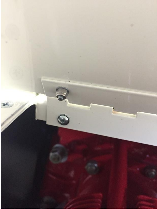
Photo 6: New Left Forward Cowl Attachment
